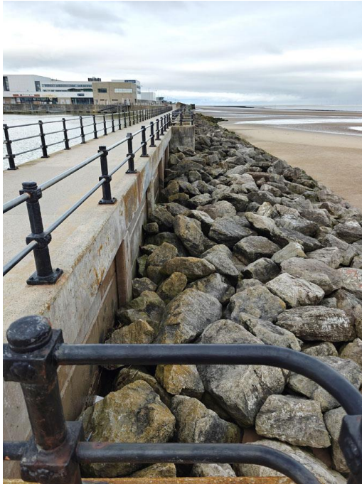
Photograph 1: Boulder Sea Defences along the Northern Impounding Wall.
