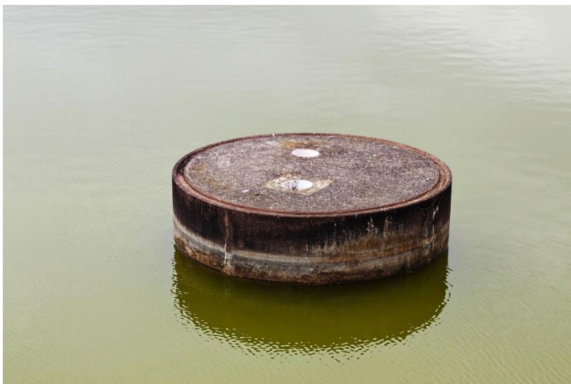
Photograph 10 overflow structure in south-east corner of the lake.
