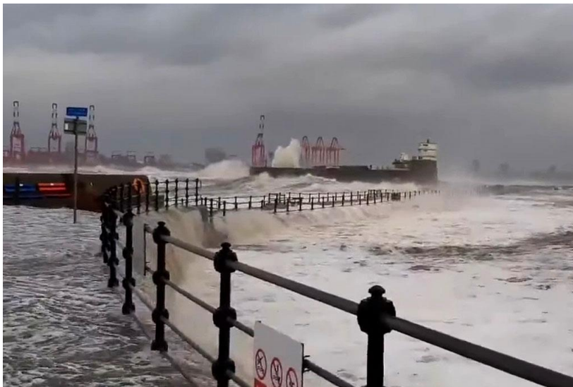
Photograph 9: Storm driven seawater inundation of the marine lake.
