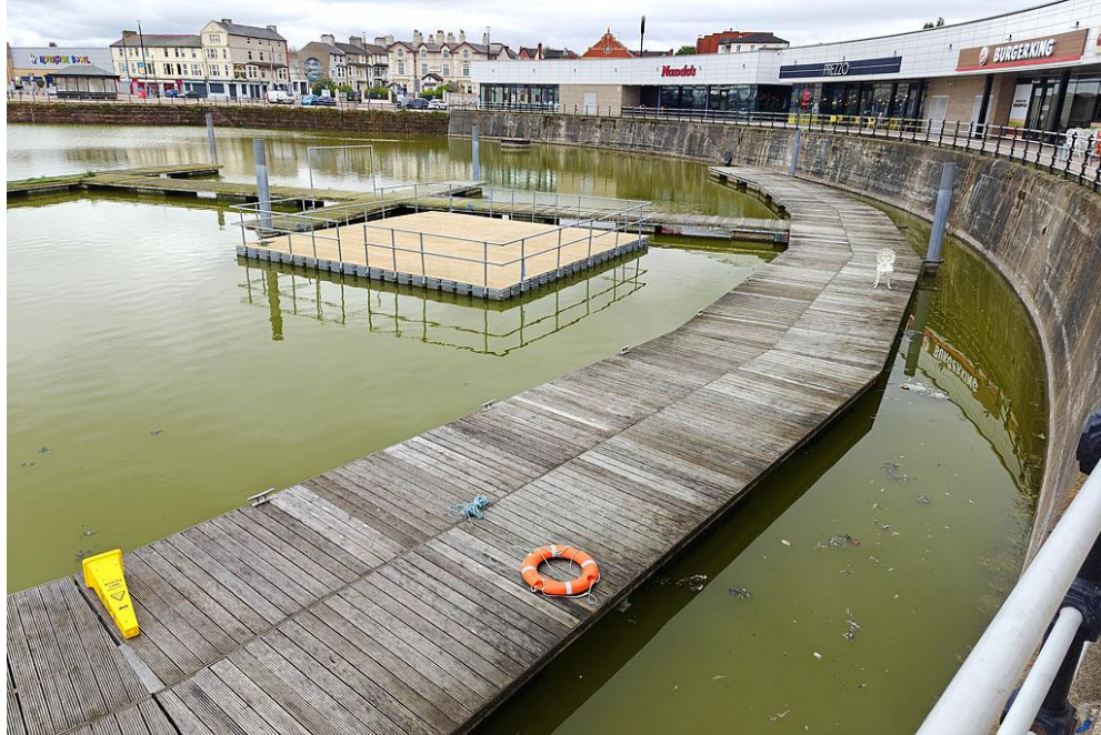
Photograph 11: Floating pontoon at the eastern end of the lake.
